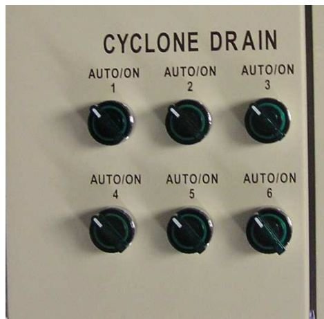
Figure 5-23 Manual Cyclone Drain Switches
